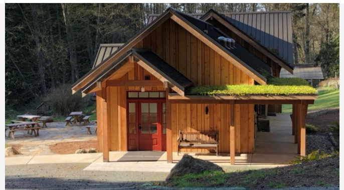
Staff install a living roof on the newly constructed commons building at the Whidbey Institute in 2021.
